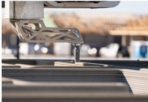
Figure 4: Example of 3D printing nozzle
