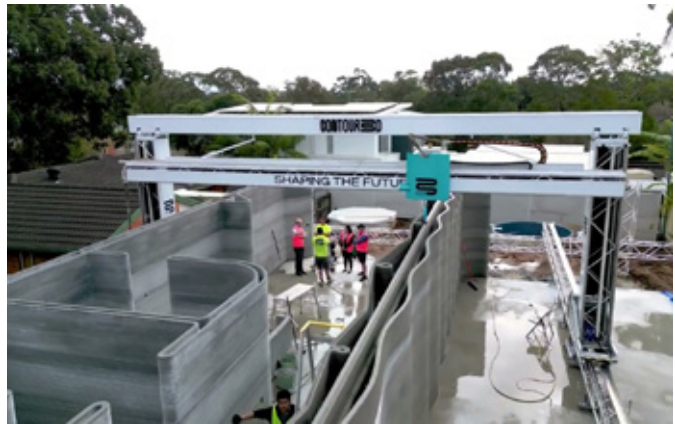
Figure 2: Full rig of the Contour3D printer
