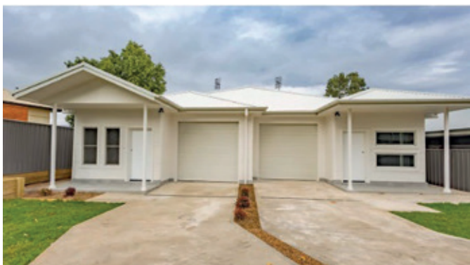
Figure 1: An example of a 3D printed home in New South Wales
