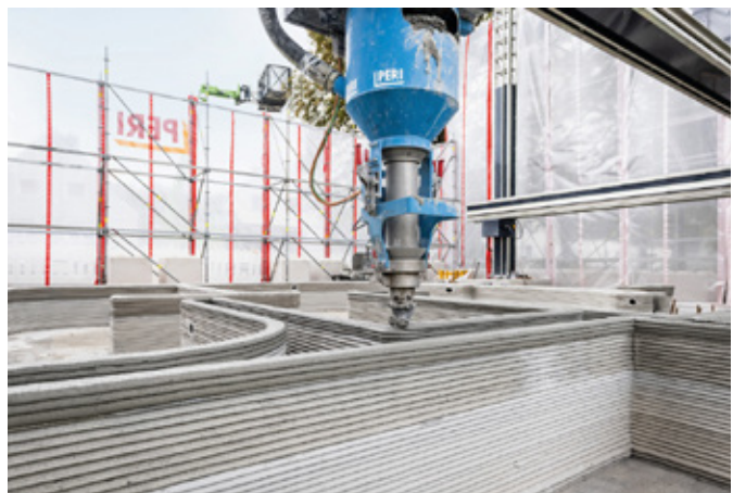
Figure 3: Concrete 3D printer in action
