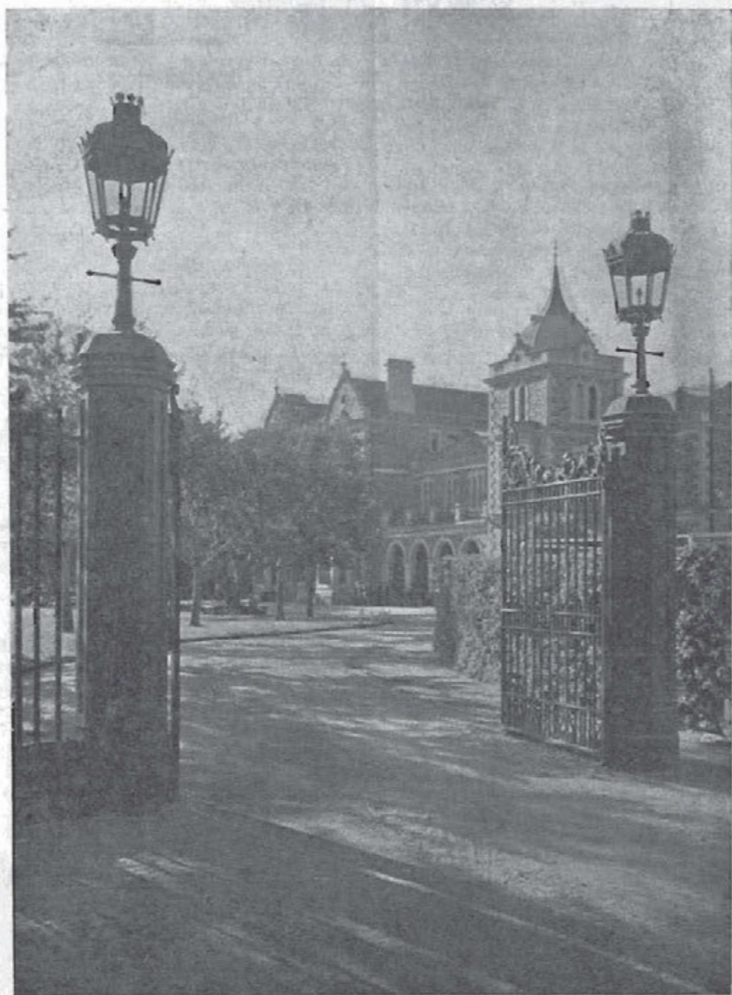
VIEW OF THE COLLEGE FROM THE GATES
