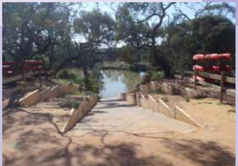
Canoe Access Ramp.
