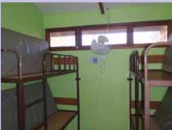
Below: Dorm 2–Painted and with new wall mounted fan.
